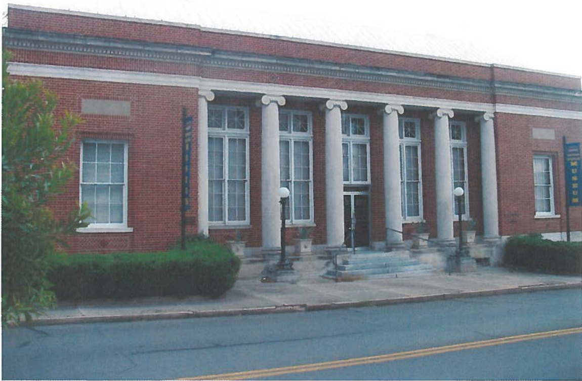
View of front façade (west side) of building.
